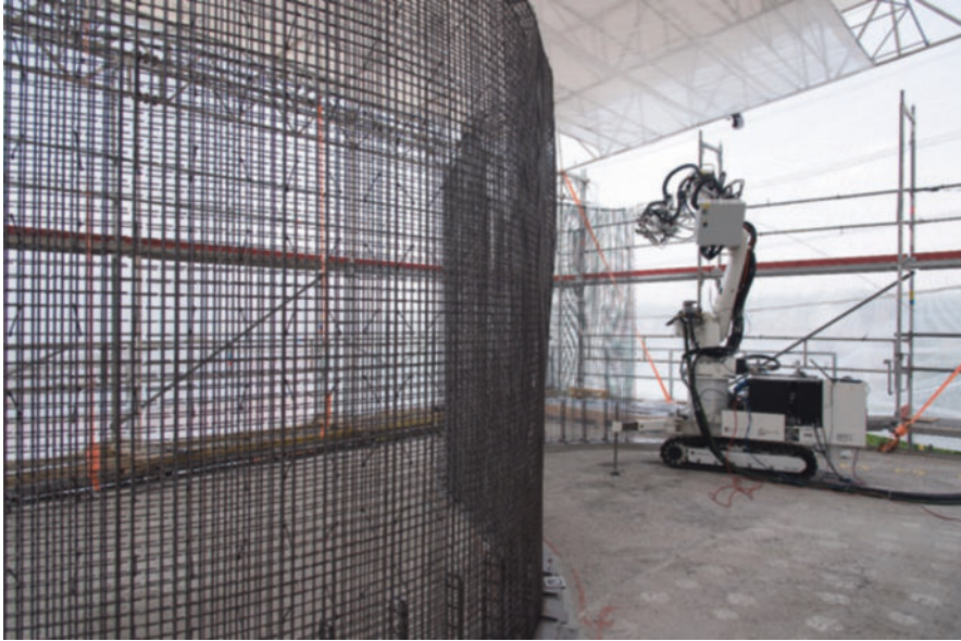
Fig. 1 The in situ fabricator building the mesh mould at the NEST house. The mesh mould process unifies the reinforcement and formwork production into a single and robotically controlled on-site fabrication system. (Image courtesy: NCCR Digital Fabrication)
