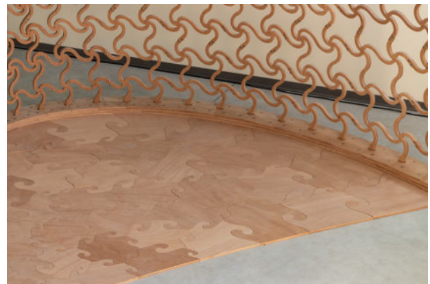
Figure 5: Variable-density interlocking Voronoi paving tiles.
