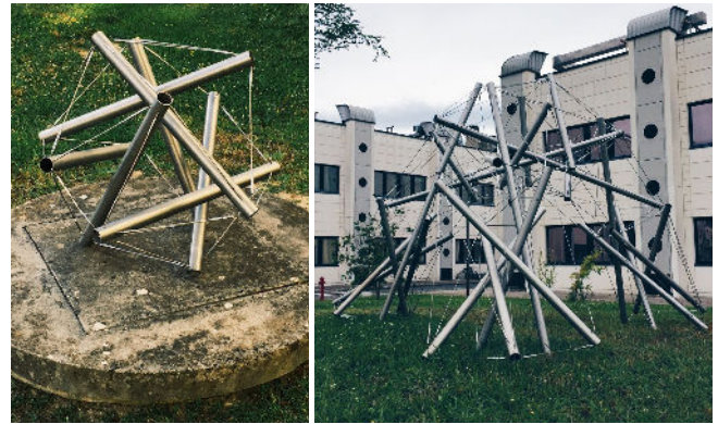
Fig. 5. Two physical tensegrity models constructed from our designs using 60 mm wide stainless steel tubes and 4 mm wide steel cables. Left: a spherical design featuring 7 struts, which is a non-trivial asymmetric variation of the popular icosahedron-based 6 struts tensegrity. Right: realization of the design shown in Figure 7-(b); see also Figure 14 and the attached video.
