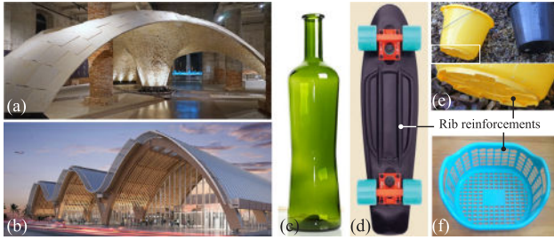
Fig. 2. Examples of shell structures showing variable thickness walls and ribs: (a) The Armadillo Vault, Biennale d'architecture 2016, has thicknesses varying from 5cm to 15cm (image by Jean-Pierre Dalbéra [2016]); (b) Mactan Cebu International Airport, Philippines (image by Denzeldoorn [2019]); (c) glass bottle of variable thickness (image by Dmitry Makeev [2006]); (d) plastic skateboard weighs 1.75kg and supports 100kg (image by MthwGlm [2020]); (e) plastic pails (image by Davie Bicker [2019]); (f) plastic laundry basket (image by Dodger67 [2013]).
